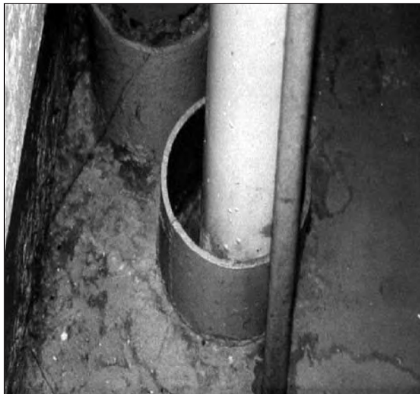
Figure 4-29 Typical conduit penetration
