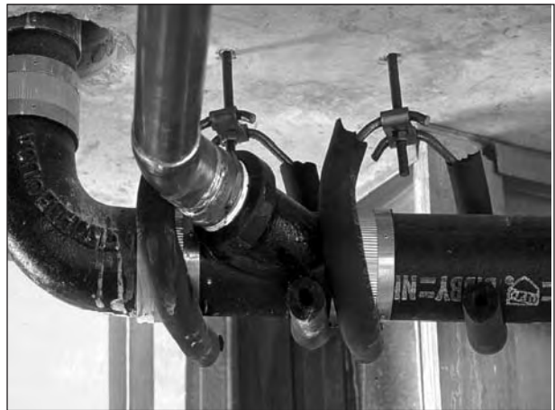
Figure 4-13 Plumbing penetrations
