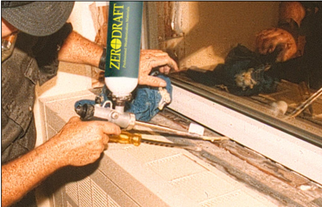
Zerodraft Foam Sealant being applied to seal gap between window frame and rough opening.
