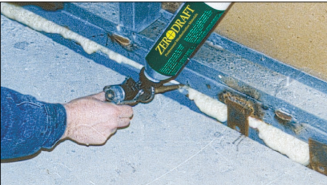
Zerodraft Foam Sealant being applied to base of wall.
